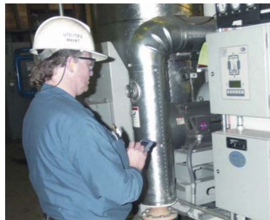
Tradesman collecting readings using Ivara EXP reliability software on handheld device - with instantaneous feedback on alarm conditions.
