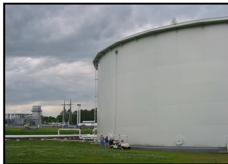
NDE wall thickness inspection, TVA Gallatin Fuel Storage Tank, 2.5 hrs including setup
